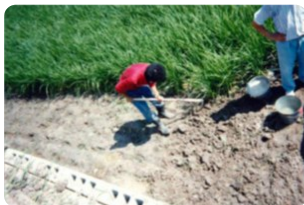
Digging up the soil and mixing in the agent
